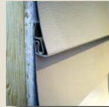
Unsupported vinyl siding (left) appears curved, while fully-supported siding with Fullback Siding Insulation (right) looks more like real wood.
